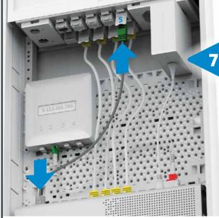
Connect the phone to a network port. Use the telephone cable to connect the «phone» port on the Internet-Box to the corresponding network port.
